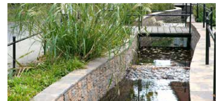
Introduction of rain gardens or swales next to a concrete encased stormwater channel
